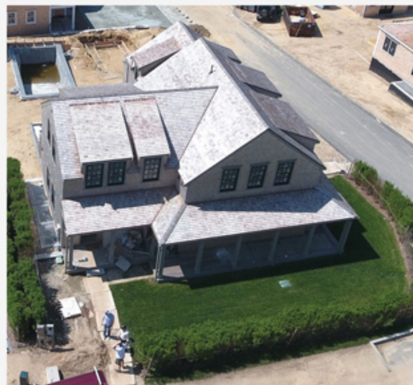
TOWN 2 Old Mill Court $3,395,000
