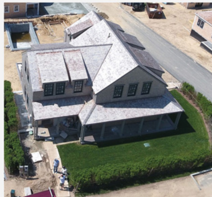
TOWN 2 Old Mill Court $3,395,000
