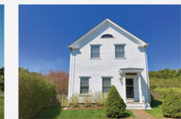
NAUSHOP 2 Dovekie Court $1,175,000
